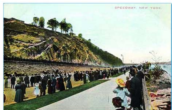
Urban helped stabilize the rock wall shown in this turn of the century engraving of the fashionable promenade along the Harlem River Speedway near High Bridge.
